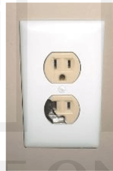
Outlet damaged.
